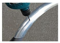
Drill the holes for the fender stay bolts through fender and mudflap. If your fender already has holes, redrill the holes (5 mm drill) through the mudflap.
